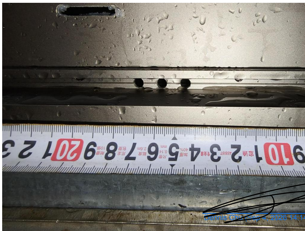
Figure 12 Photo of Weep Holes Detail
