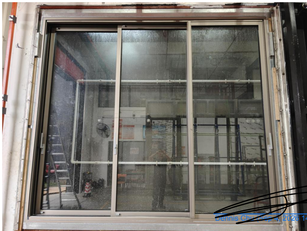
Figure 12 Photo of Test Specimen Closed (Interior) After Test
