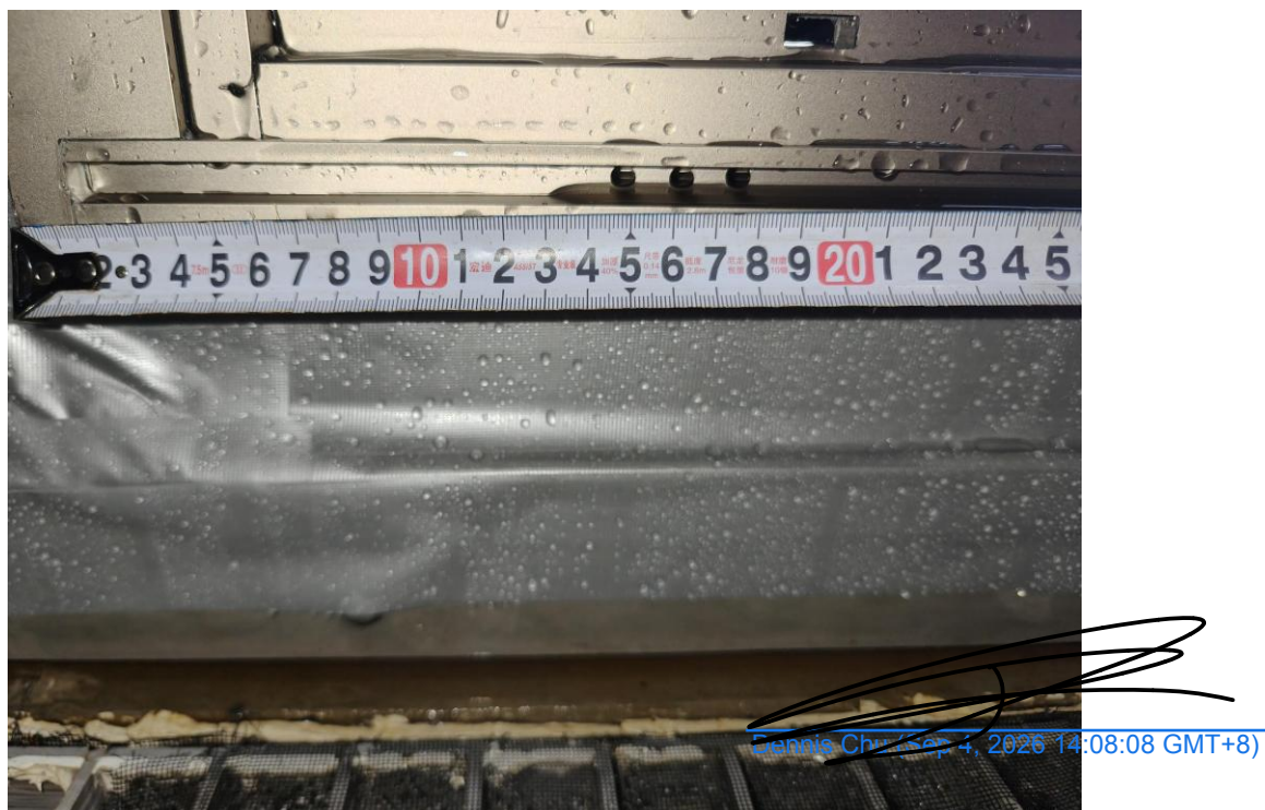
Figure 11 Photo of Drainage / Weep Holes Detail
