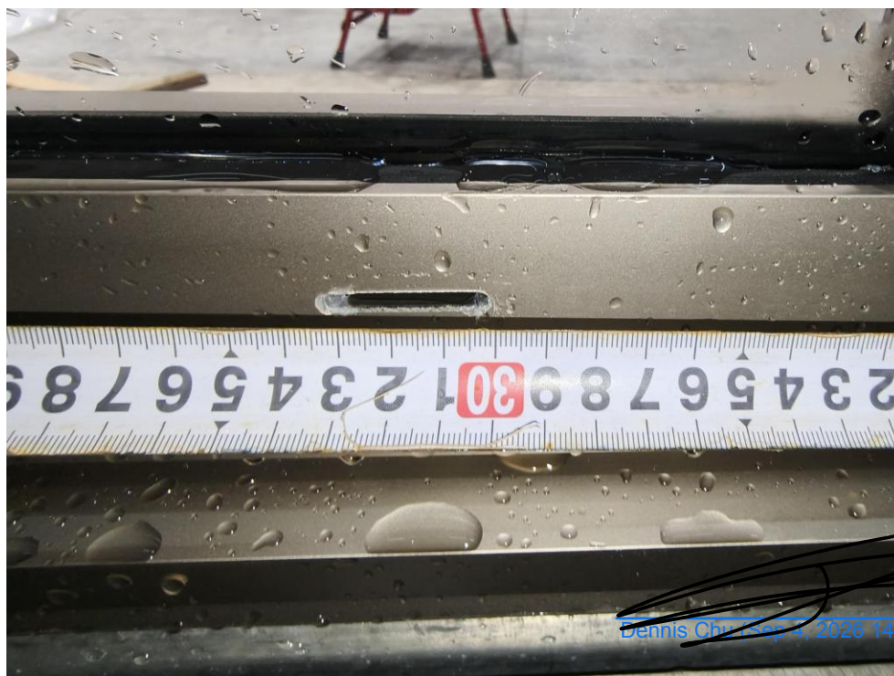
Figure 10 Photo of Drain Holes Detail
