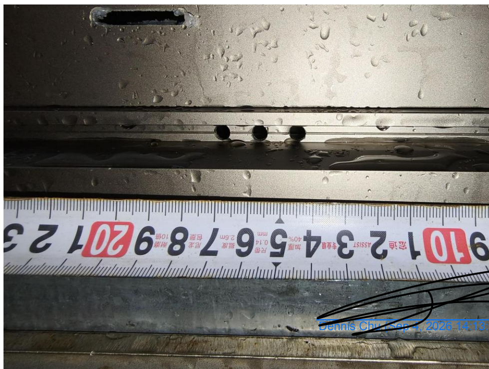
Figure 12 Photo of Weep Holes Detail
