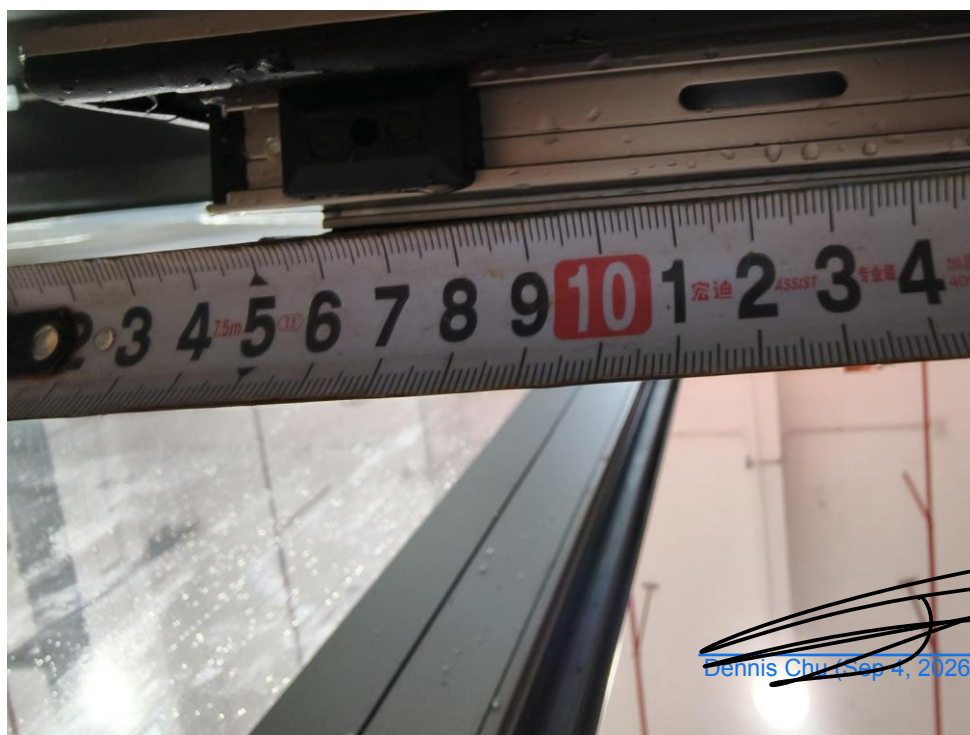
Figure 11 Photo of Drain Holes Detail
