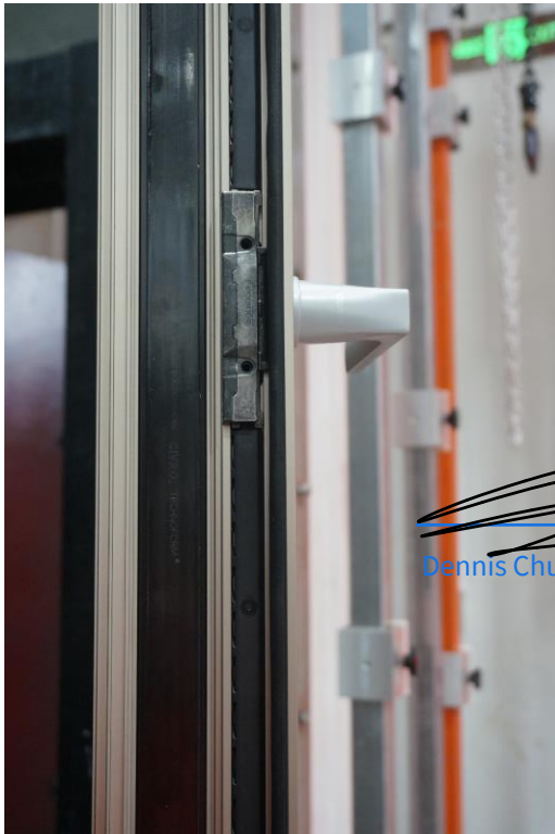
Figure 11 Photo of Hardware (Handle and Blot)
