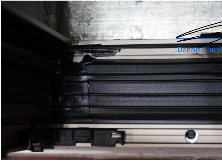
Figure 16 Photo of Tilt-turn Lock bracket and Support Base
