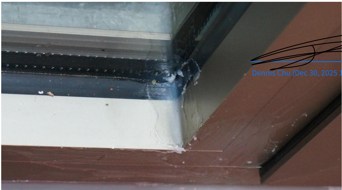
Figure 9 Connection Detail Between Right Side Jamb and Bottom Rail (Showing White Traces Left by Transparent Waterproof Coating on Surface)
