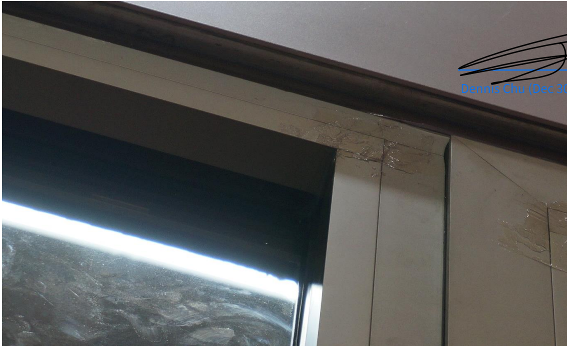
Figure 4 Connection Detail Between Interlock Stile and Two Panels 1 (Showing White Traces Left by Transparent Waterproof Coating on Surface)
