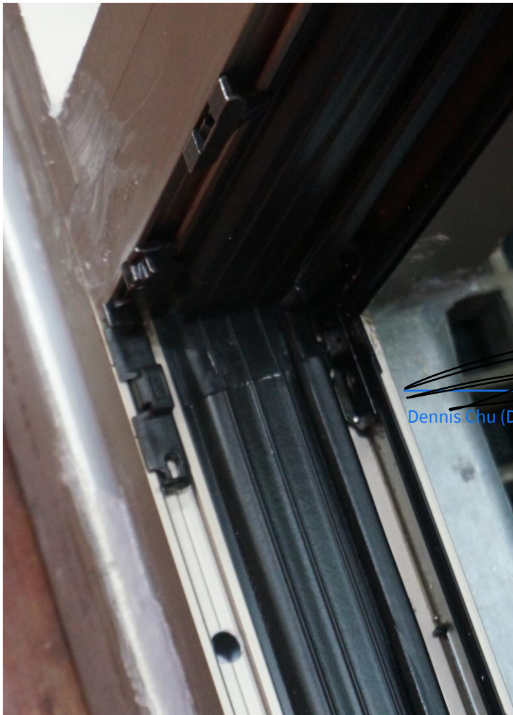
Figure 17 Photo of Tilt-turn Lock bracket and Support Base (Zoom in)
