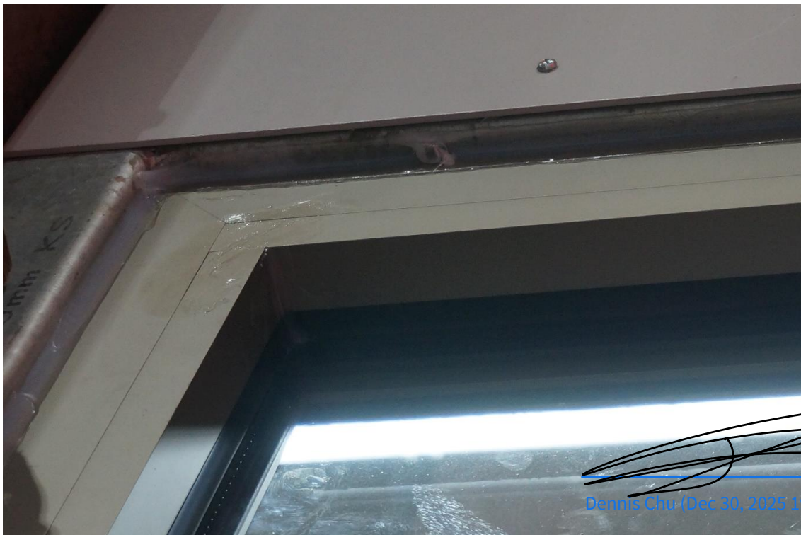
Figure 7 Connection Detail of Left Side Jamb, Head Jamb, and Fixed Panel (Showing White Traces Left by Transparent Waterproof Coating on Surface)
