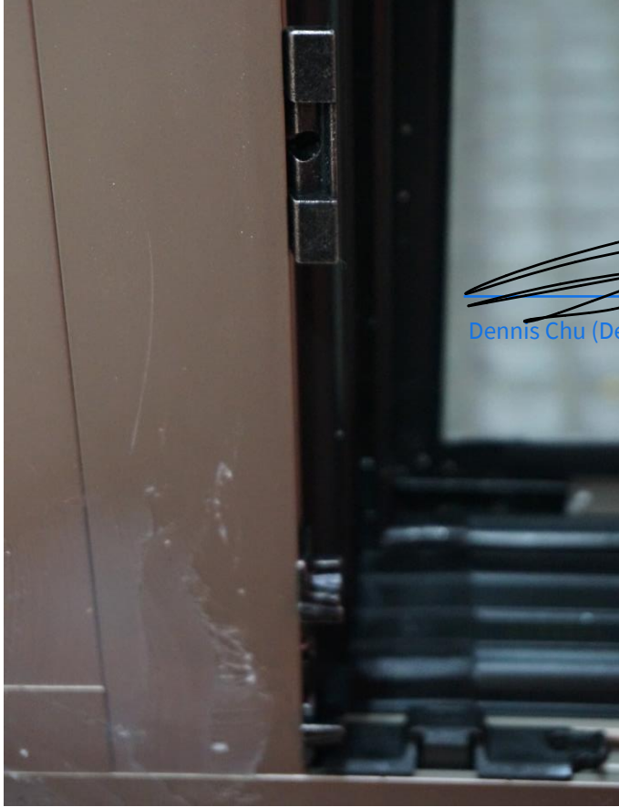
Figure 18 Photo of Standard Lock bracket
