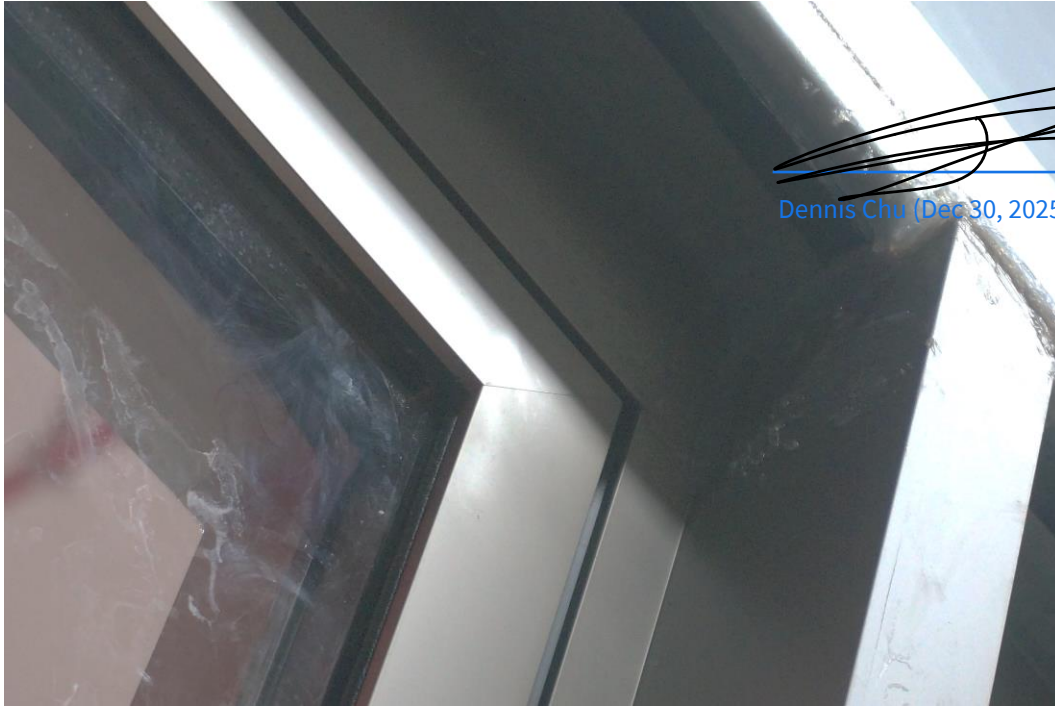
Figure 26 Connection of Mullion and Head 1 (View from Exterior)
