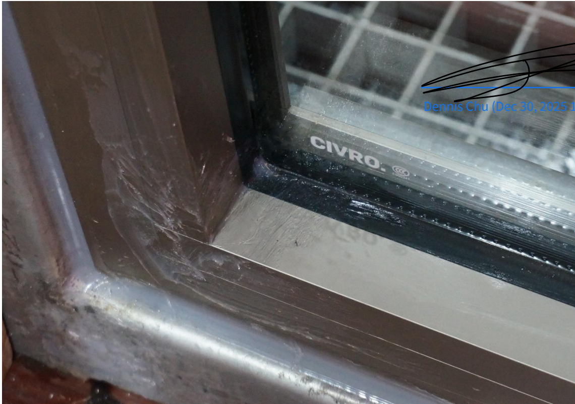
Figure 8 Connection Detail Between Left Side Jamb and Bottom Rail (Showing White Traces Left by Transparent Waterproof Coating on Surface)
