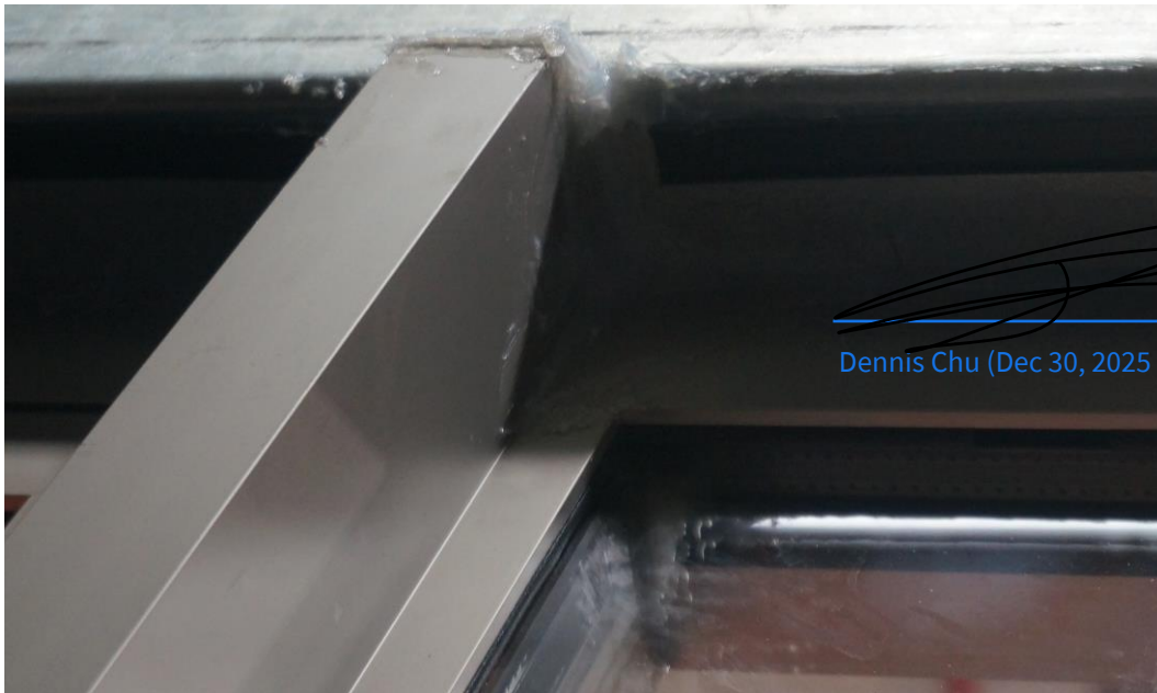
Figure 27 Connection of Mullion and Head 2 (View from Exterior)
