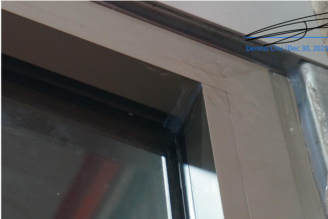
Figure 6 Connection Detail of Right-Side Jamb, Head Jamb, and Operable Sash (Showing White Traces Left by Transparent Waterproof Coating on Surface)
