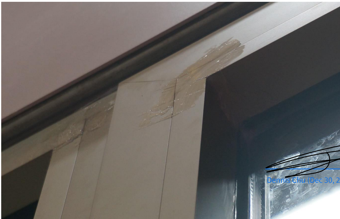
Figure 5 Connection Detail Between Interlock Stile and Two Panels 2 (Showing White Traces Left by Transparent Waterproof Coating on Surface)
