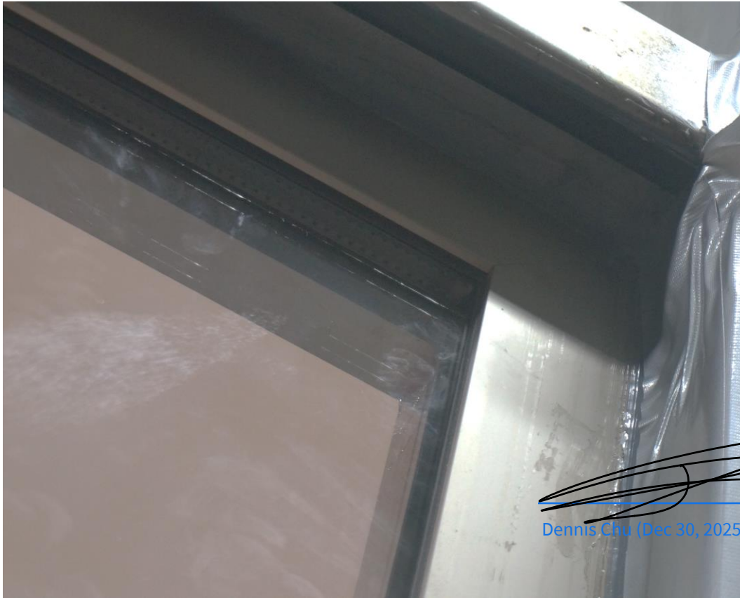
Figure 28 Photo of Outer Frame Top Right Corner (View from Exterior)
