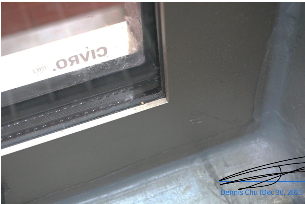
Figure 29 Photo of Outer Frame Top Right Corner (View from Exterior)
