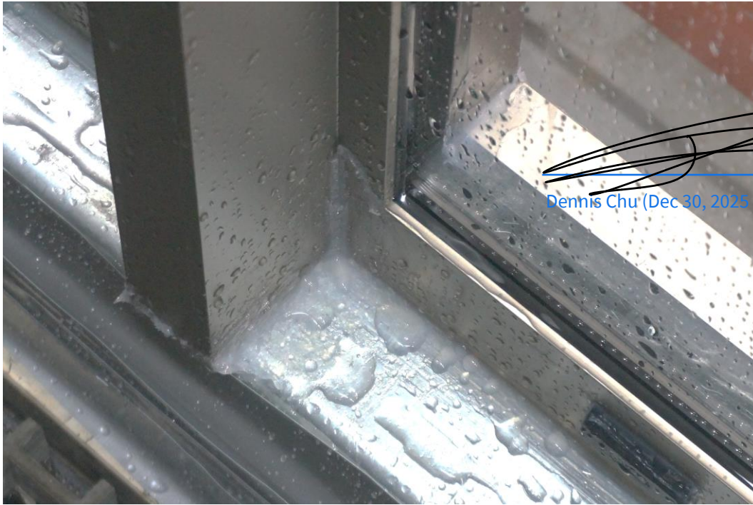
Figure 24 Connection of Mullion and Bottom Rail (View from Exterior)
