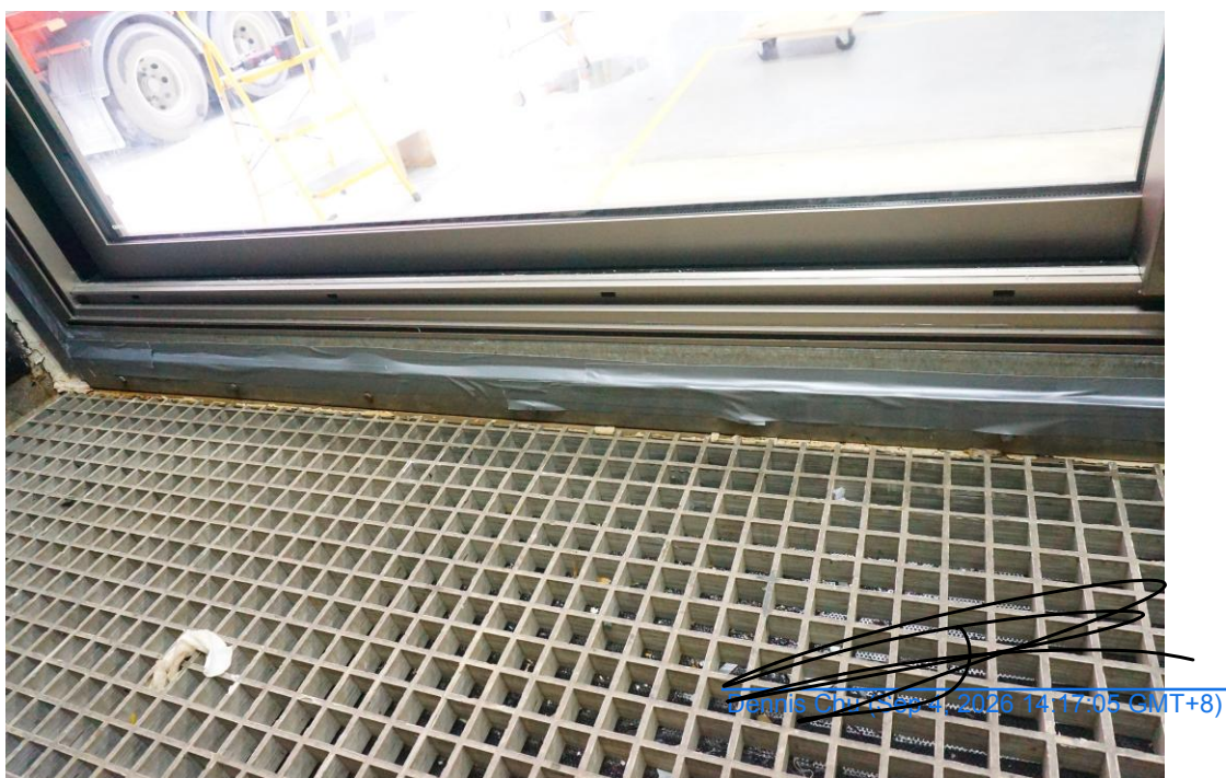
Figure 11 Photo of Drain Holes Detail
