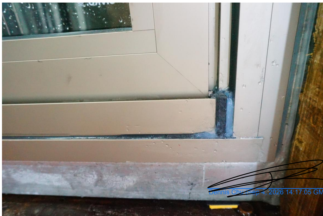
Figure 13 Photo of Joint
