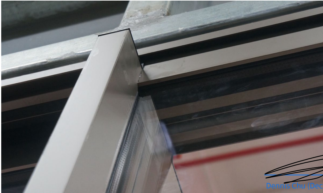
Figure 18 Connection Detail Between Two Panels
