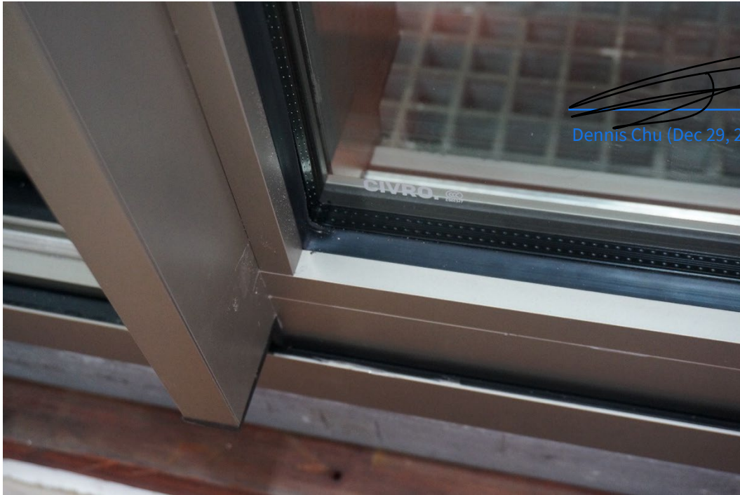
Figure 10 Connection Detail Between Bottom Sill, Interlock Stile, Door Track, Bottom Rail and Right Panel (Showing White Traces Left by Transparent Waterproof Coating on Surface)
