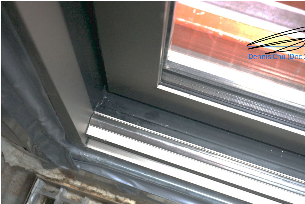
Figure 15 Connection Detail Between Bottom Sill, Lock Stile, Door Track, Bottom Rail and Jamb (View from Exterior)
