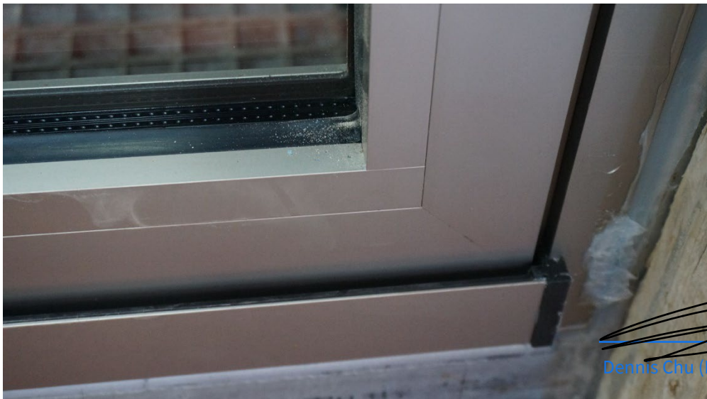
Figure 11 Connection Detail Between Right Side Jamb, Bottom Sill, Bottom Rail and Right Lock Stile (Showing White Traces Left by Transparent Waterproof Coating on Surface)
