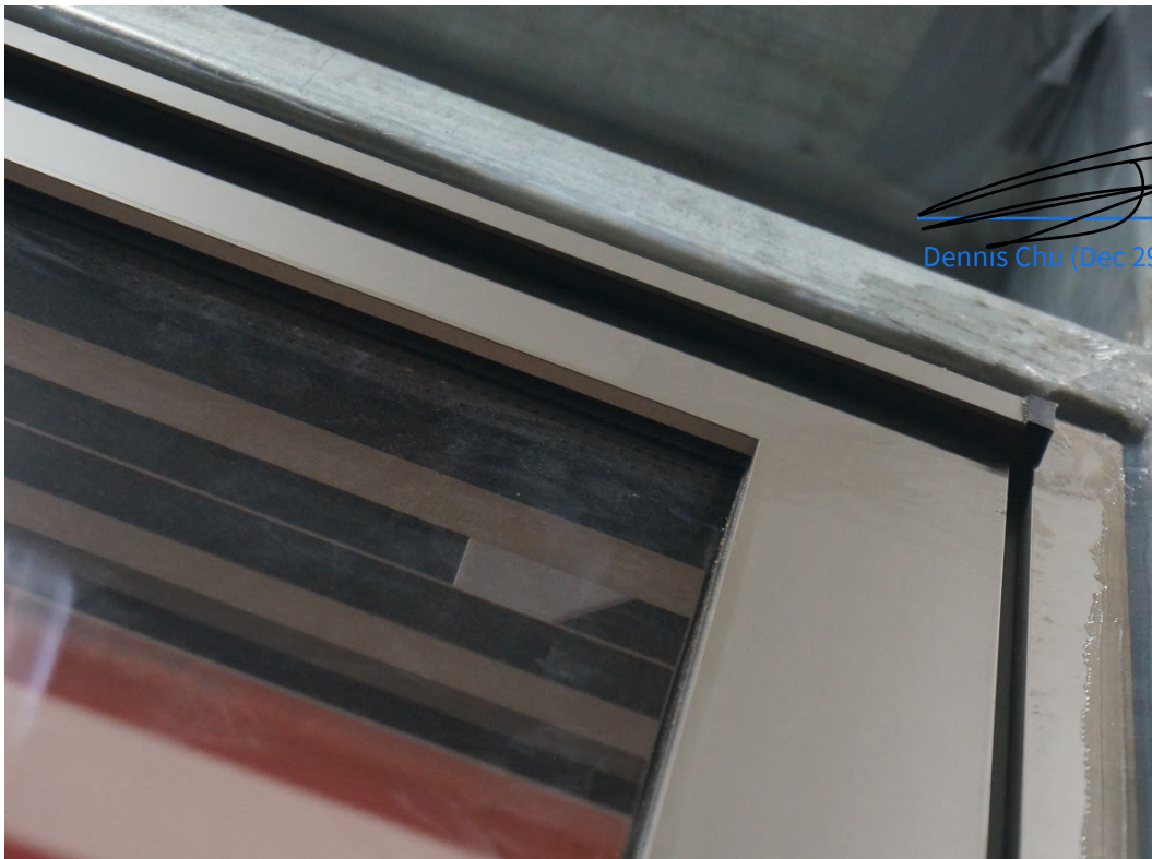
Figure 19 Connection Detail Between Top Rail, Lock Stile, Door Track, Bottom Rail and Right-Side Jamb (View from Exterior)
