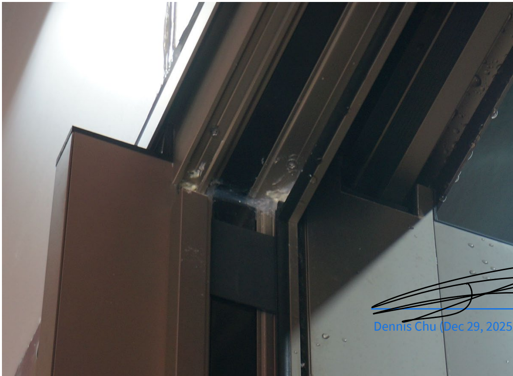
Figure 25 Connection Detail Between Head, Interlock Stile and Door Track (Right Panel)
