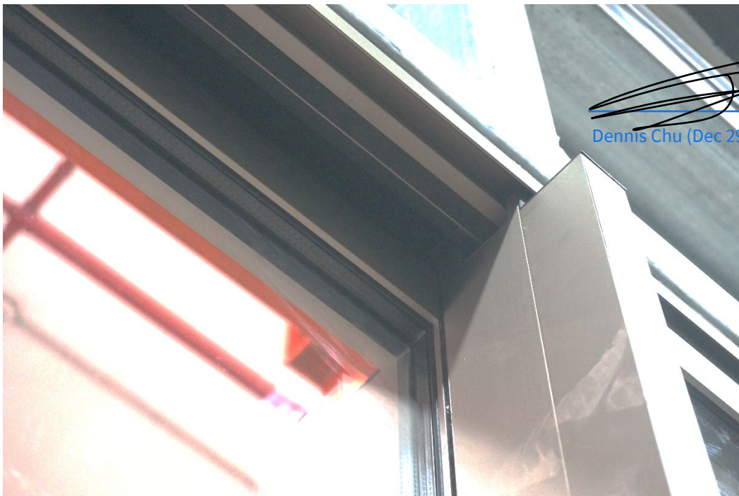
Figure 17 Connection Detail Between Top Rail, Interlock Stile and Head (Showing White Traces Left by Transparent Waterproof Coating on Surface)
