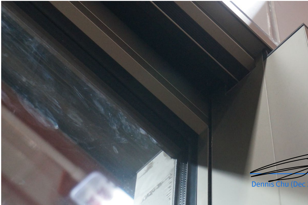
Figure 13 Connection Detail Between Head and Interlock Stile
