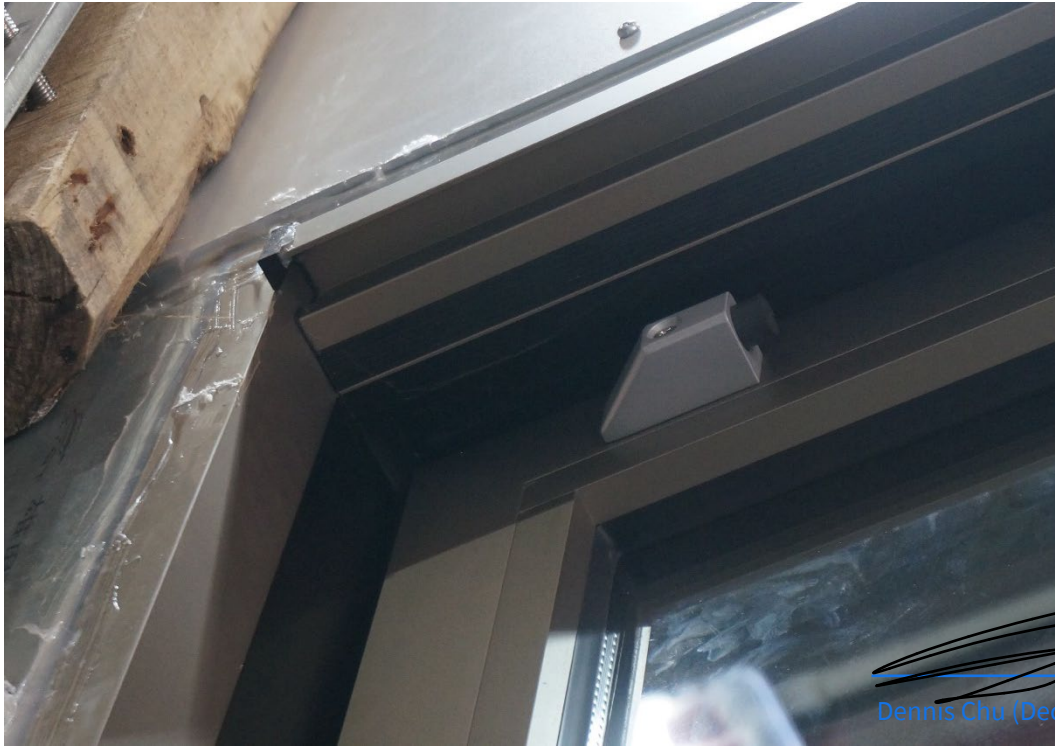
Figure 14 Door Bumper Stop Installed on Top Rail of Left Panel
