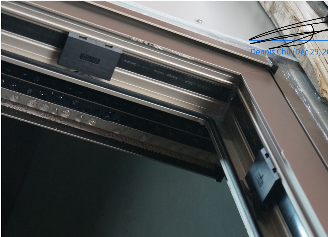
Figure 24 Connection Detail Between Head, Right-Side Jamb and Door Track
