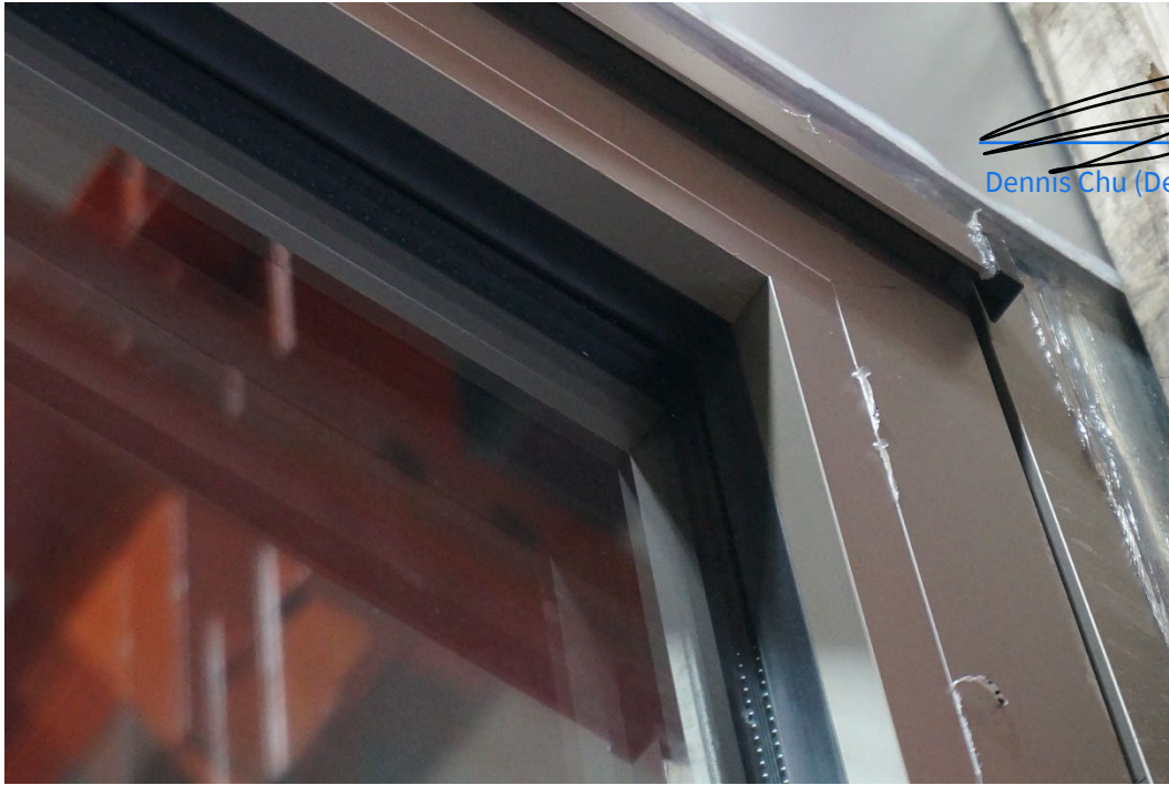
Figure 12 Connection Detail Between Right Side Jamb, Head, Top Rail, and Right Lock Stile (Showing White Traces Left by Transparent Waterproof Coating on Surface)
