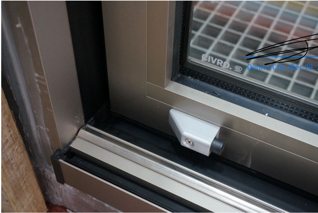
Figure 8 Connection Detail Between Left Side Jamb, Bottom Sill, Lock Stile and Bottom Rail
