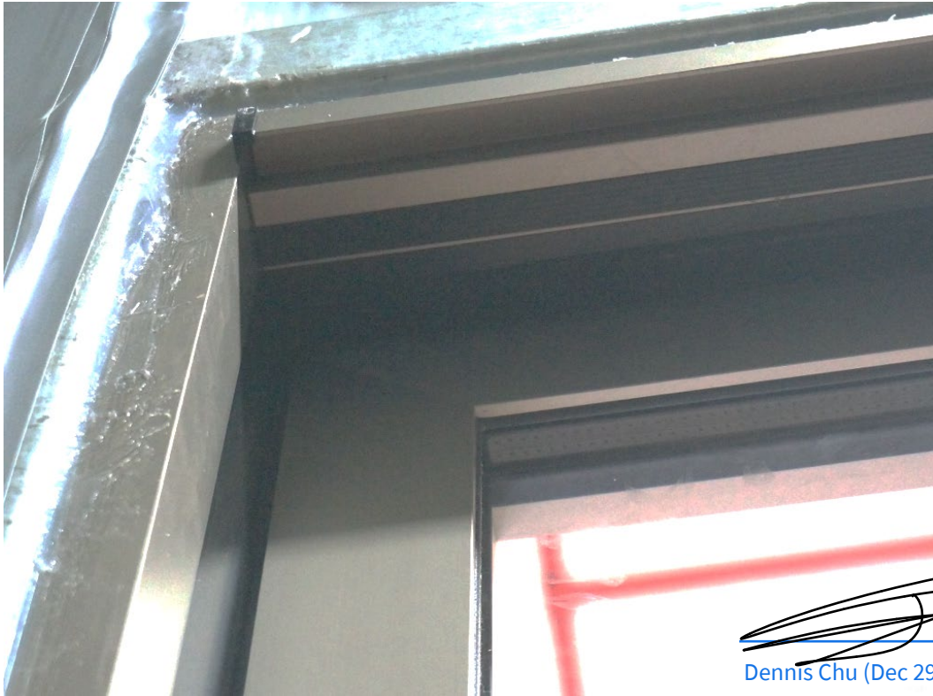
Figure 16 Connection Detail Between Top Rail, Lock Stile, Door Track, Bottom Rail and Left-Side Jamb (View from Exterior)
