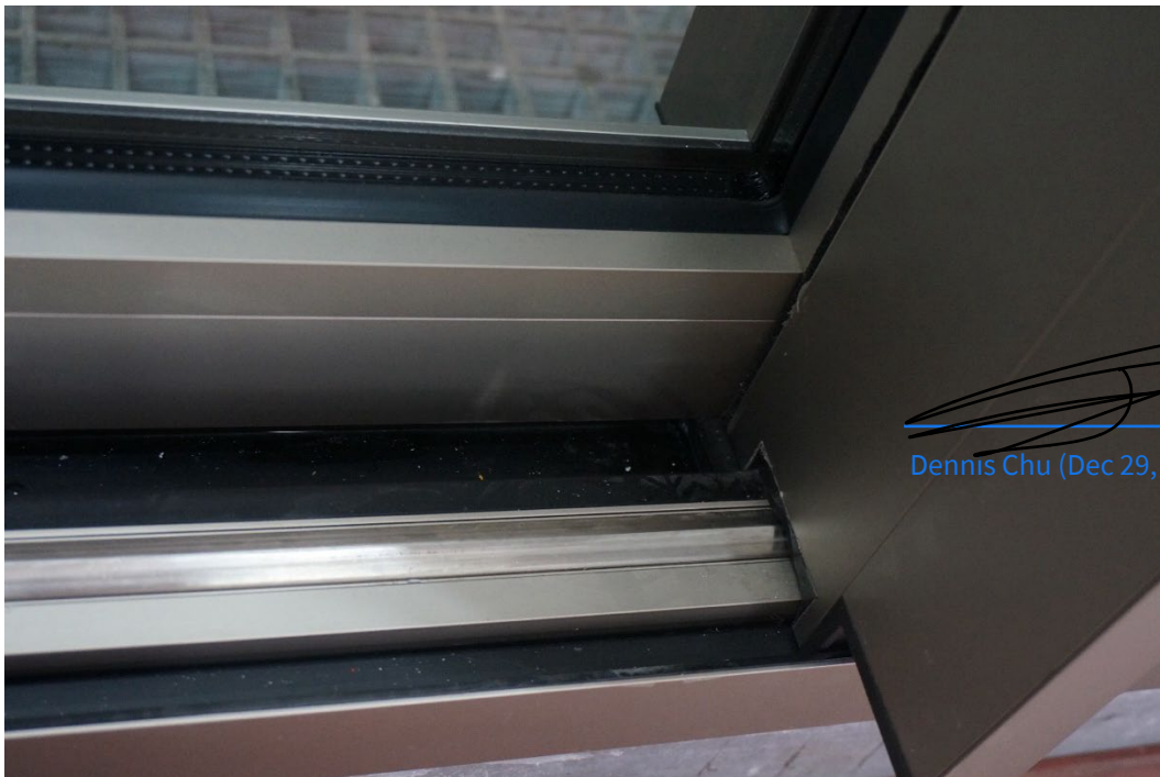
Figure 9 Connection Detail Between Bottom Sill, Interlock Stile, Door Track, Bottom Rail and Left Panel
