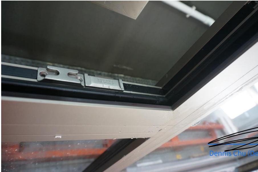
Figure 14 Photo of Locking Point and Locking Keeper (Right Side)
