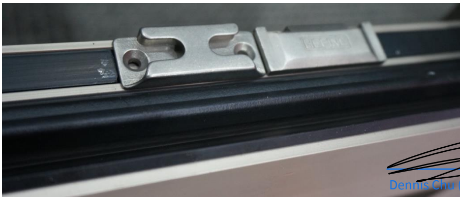
Figure 15 Photo of Locking Point and Locking Keeper (Right Side)
