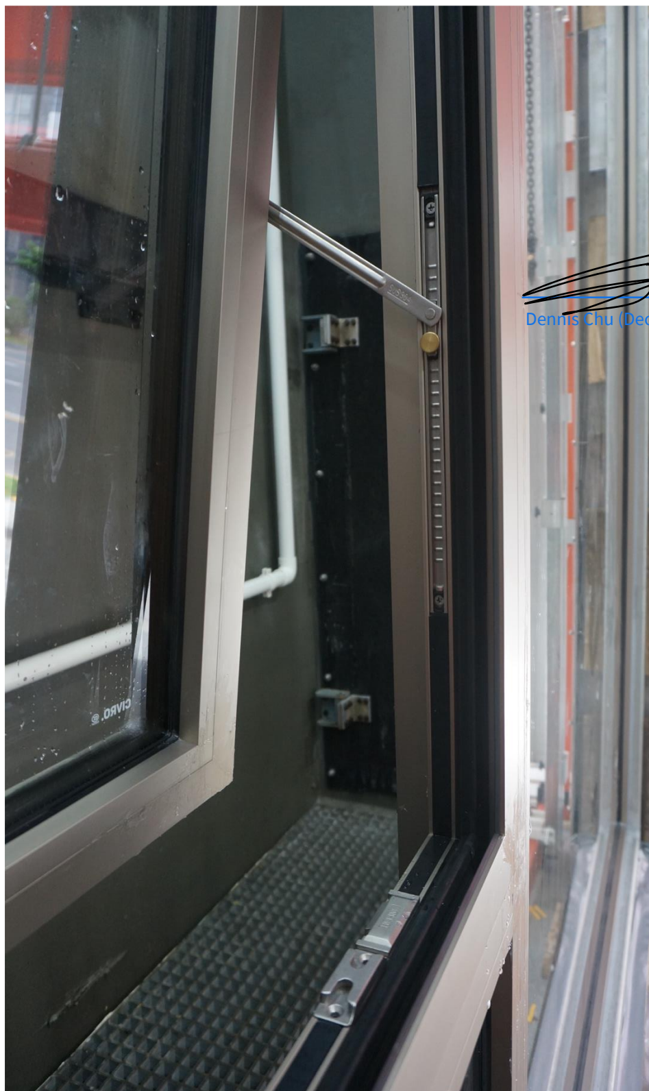
Figure 17 Awning Window in Opened Position Showing the Friction Stay Hinges, Locking Point and Keeper (Left Side)
