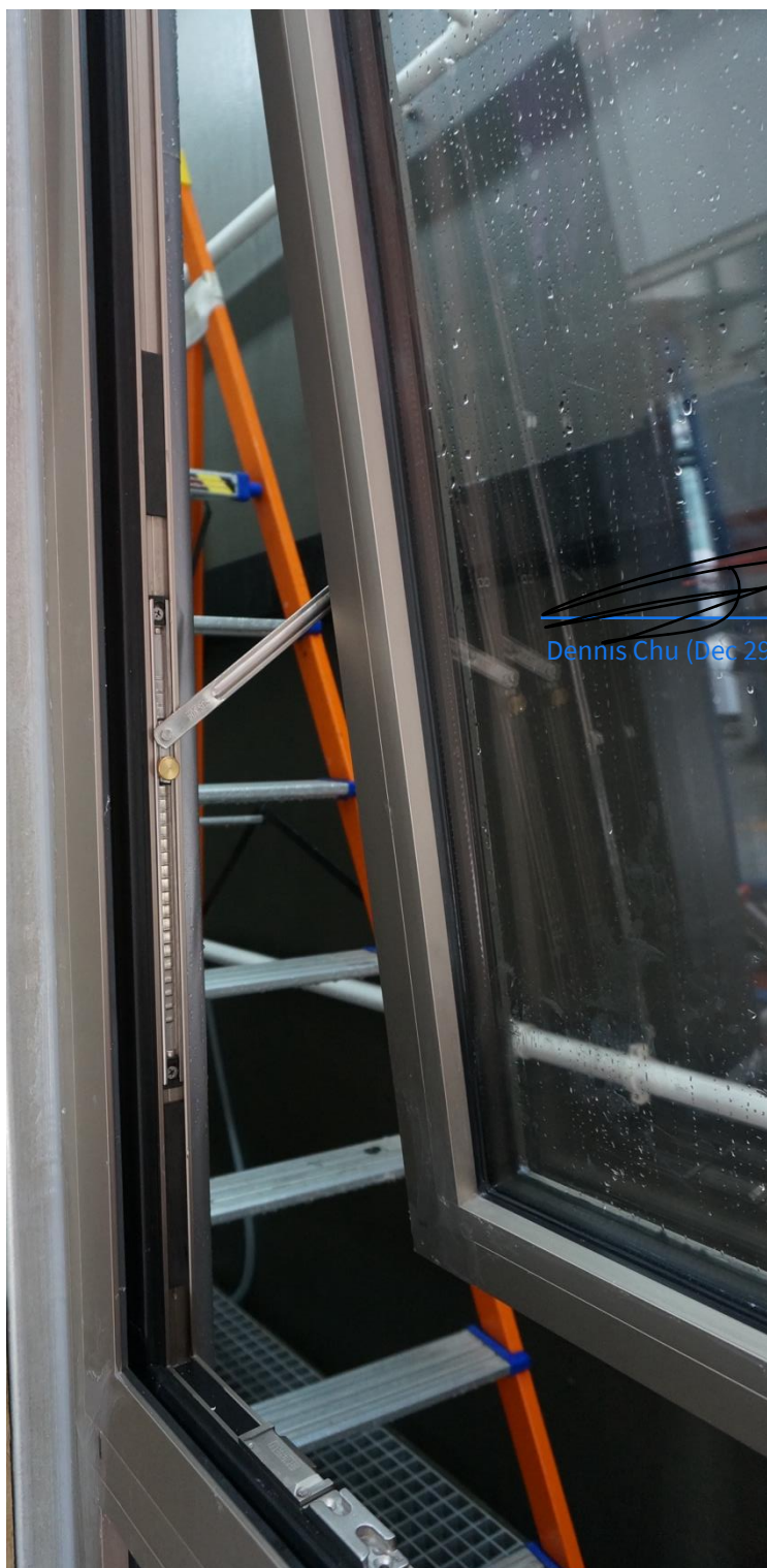
Figure 18 Awning Window in Opened Position Showing the Friction Stay Hinges, Locking Point and Keeper (Right Side)
