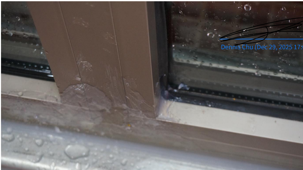
Figure 22 Connection Detail of Mullion and Bottom Sill
