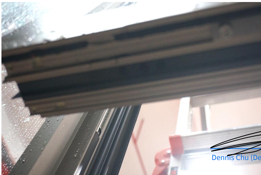
Figure 12 Photo of Bottom Rail (Taken from Bottom-to-Top Angle) Showing Weather Strip Detail
