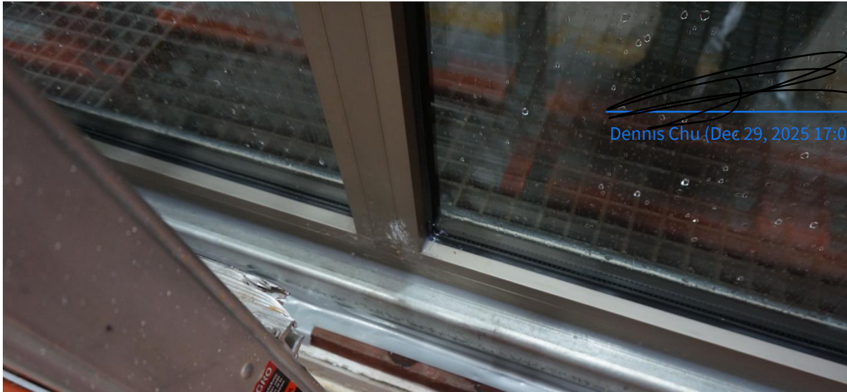
Figure 8 Connection Detail Between Mullion and Bottom Rail
