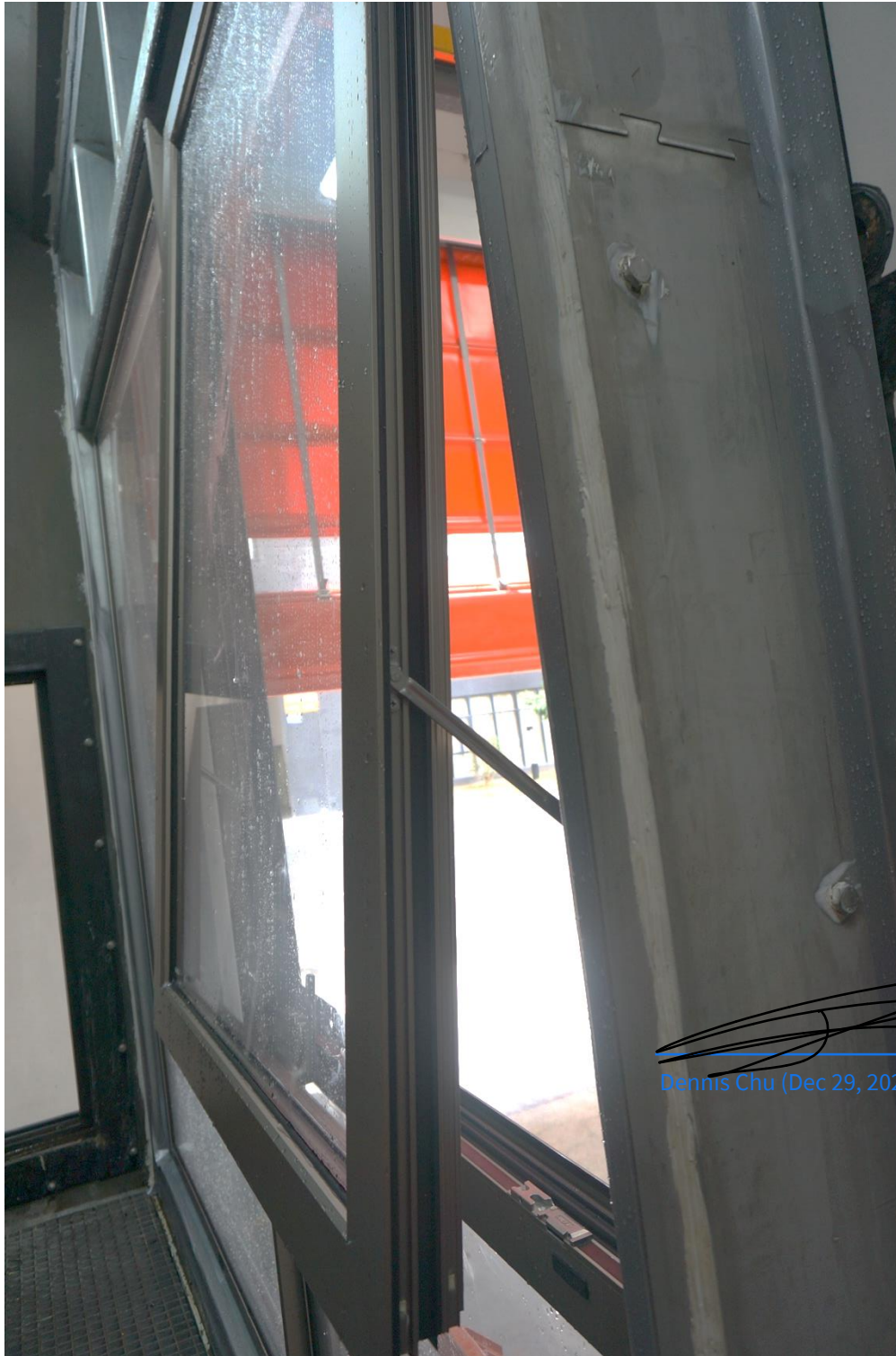
Figure 30 Photo of Operable Sash in Open Position (View from Bottom and Exterior) Showing Detail of Hardware – locking points & Limit Stay
