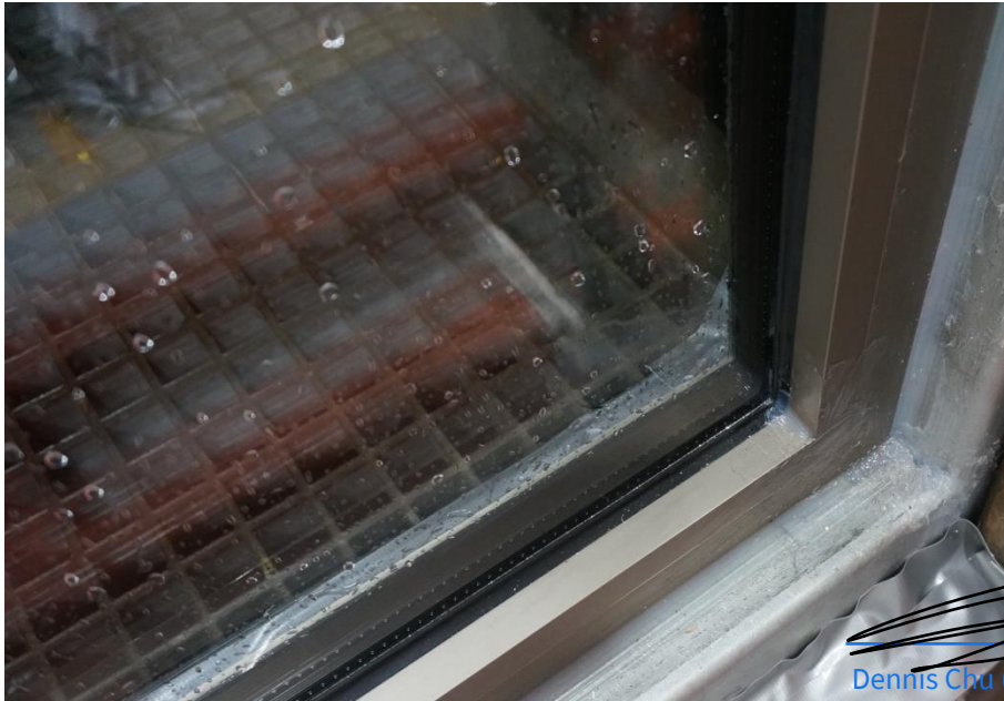
Figure 10 Connection Detail Between Right Side Jamb and Bottom Rail
