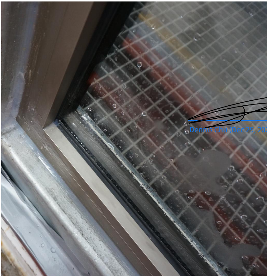
Figure 9 Connection Detail Between Left Side Jamb and Bottom Rail
