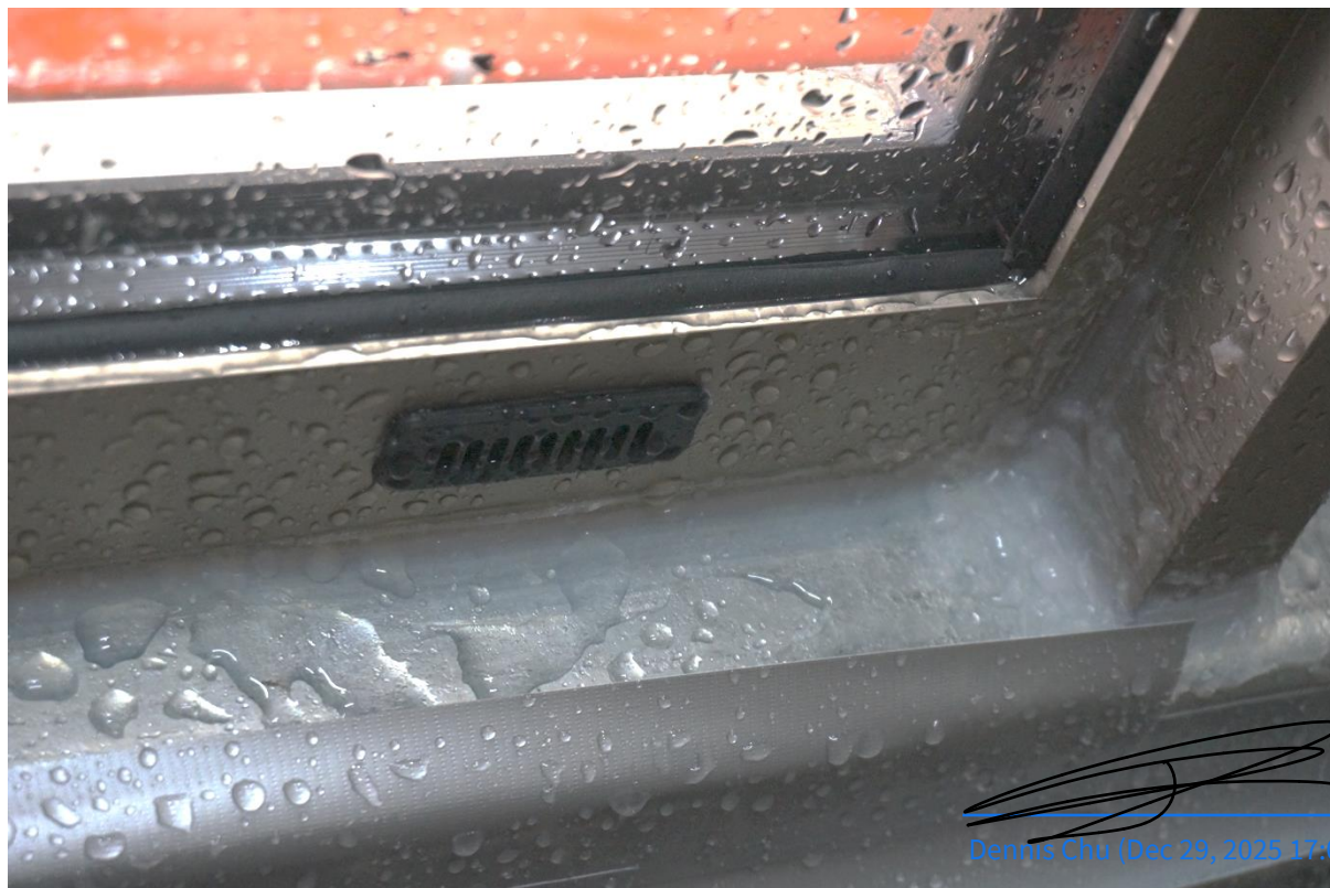
Figure 31 The Bottom Sill of Window Assembly (View from Exterior)
