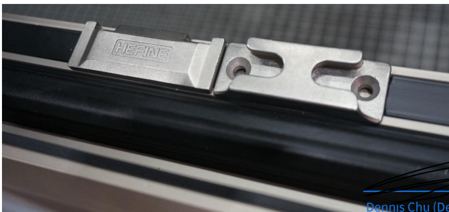
Figure 16 Photo of Locking Point and Locking Keeper (Left Side)
