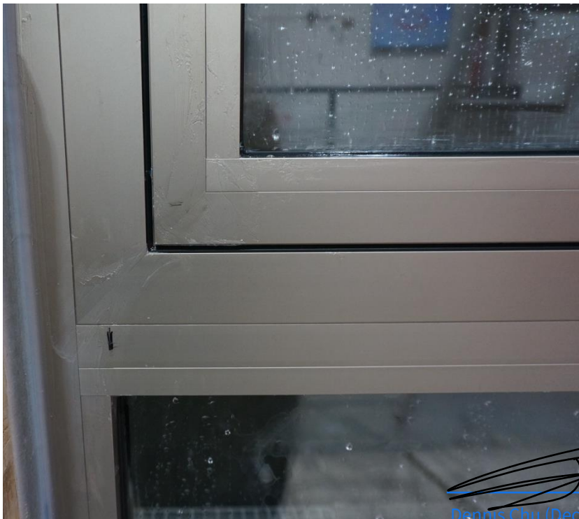
Figure 5 Connection Detail Between Operable Sash and Fixed Window (Left Side)
