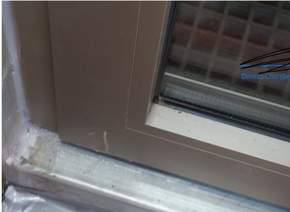
Figure 6 Photo of the Sill-jamb junction (Bottom Left corner) of the Inwards Swing Door) (Showing White Traces Left by Transparent Waterproof Coating on Surface)
