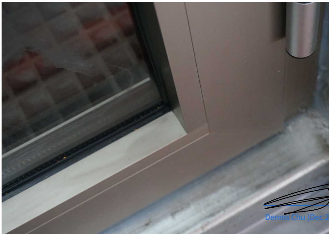
Figure 7 Photo of the Sill-jamb junction (Bottom Right corner) of the Inwards Swing Door)
