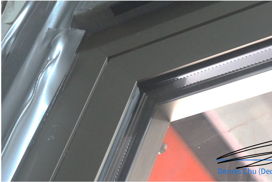
Figure 17 Photo of Top Left Corner of Door Frame, Top Rail and Stile (View from Exterior)
