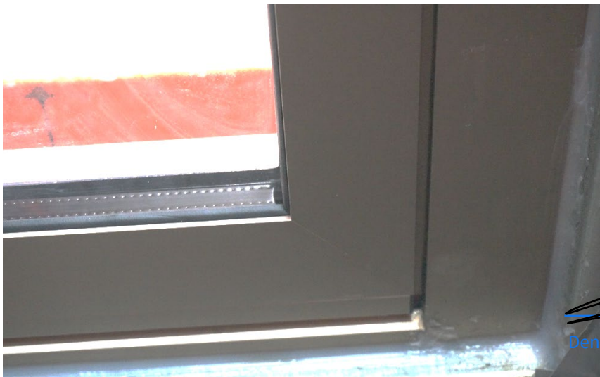
Figure 20 Photo of Bottom Right Corner of Door Frame, Bottom Sill and Stile (View from Exterior) (Showing White Traces Left by Transparent Waterproof Coating on Surface)
